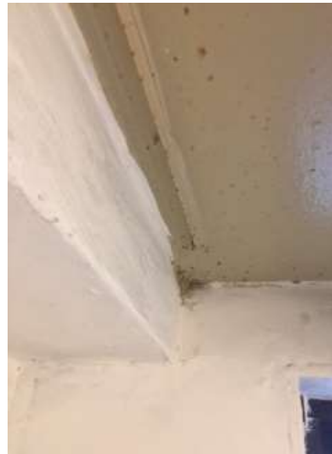
Close Up: Bathroom Ceiling
