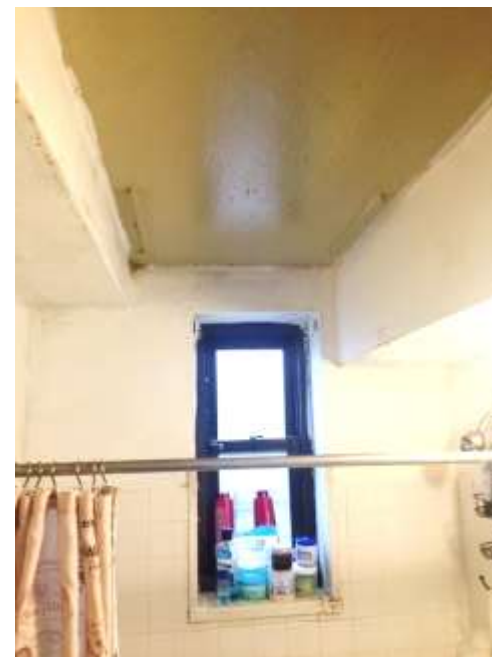
Full View: Bathroom Wall
