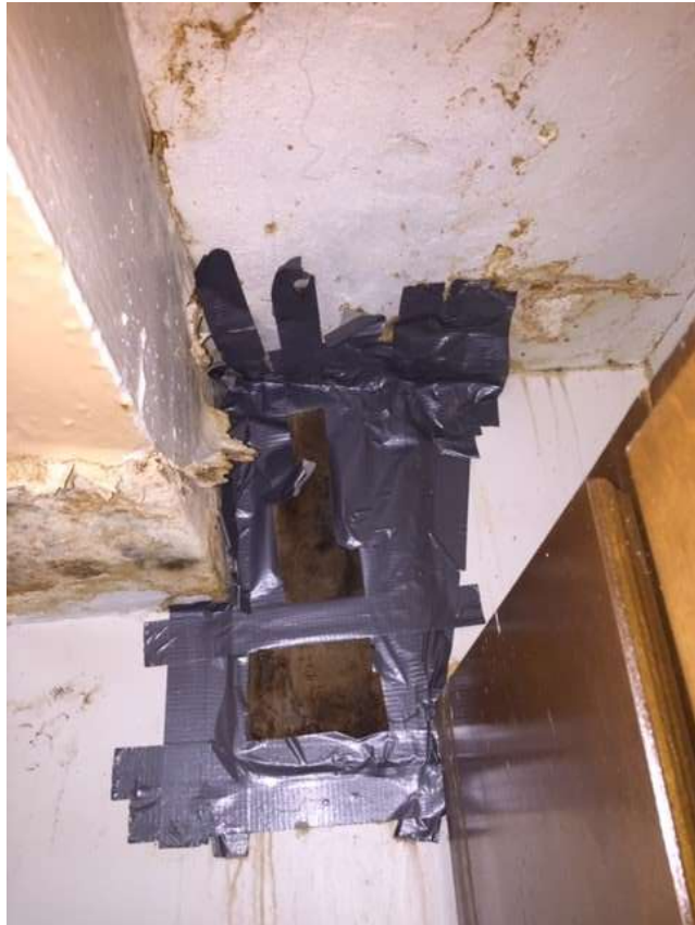
Close Up: Kitchen
