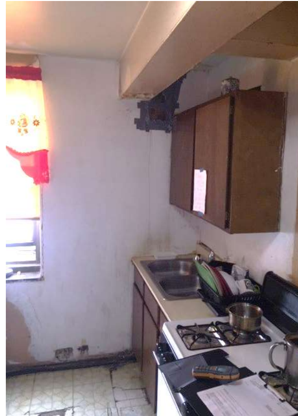
Full View: Kitchen
