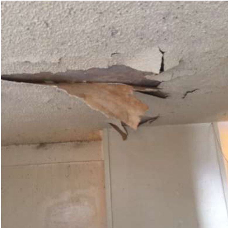
Close Up: Living Room Ceiling
