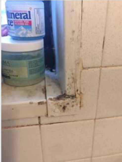
Close Up: Bathroom Window Frame
