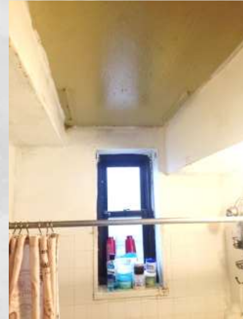
Full View: Bathroom Wall
