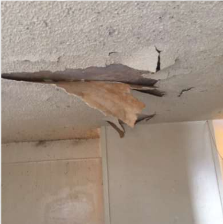
Close Up: Living Room Ceiling
