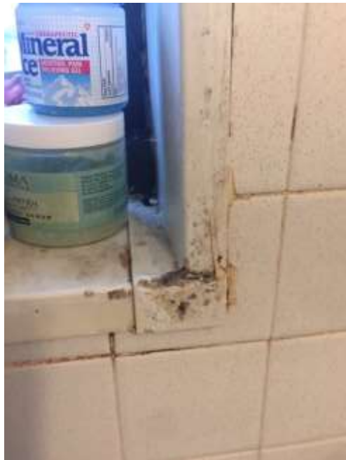
Close Up: Bathroom Window Frame
