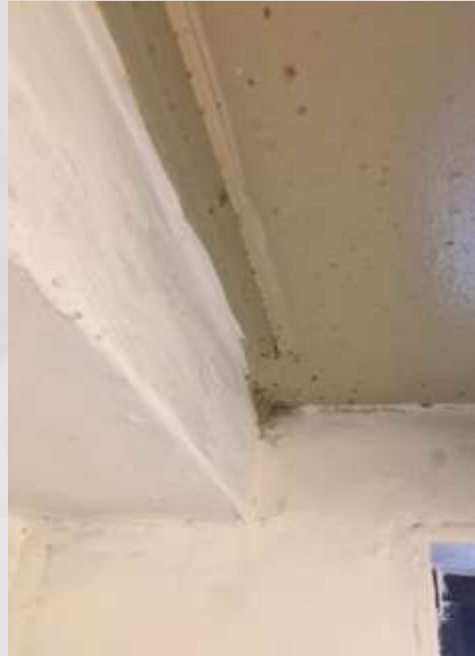
Close Up: Bathroom Ceiling
