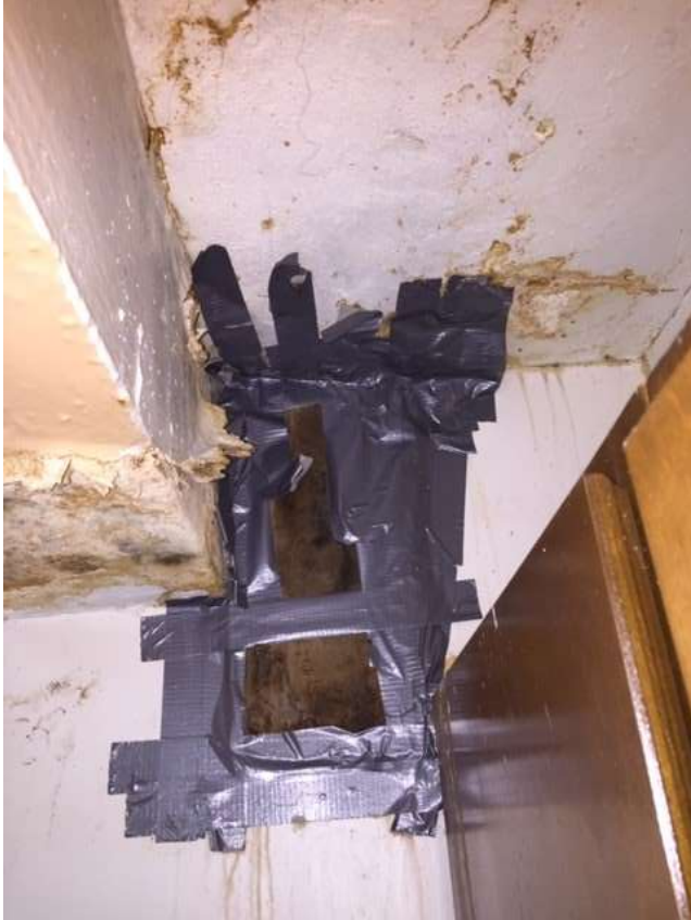
Close Up: Kitchen
